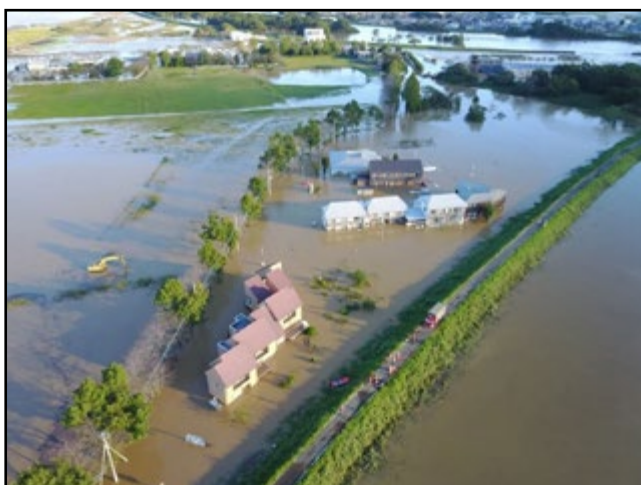
Fig. 1 Group homes and a residential facility of a social welfare cooperation for persons with severe autism, Keyaki-no-sato, Kawagoe, Japan, had flooded in 1999 and 2019.
