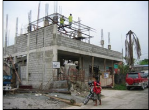
The construction of a new and accessible office and training facility for the National Federation of Cooperatives of Persons with Disabilities (NFCPWD) in Metro Manila.
